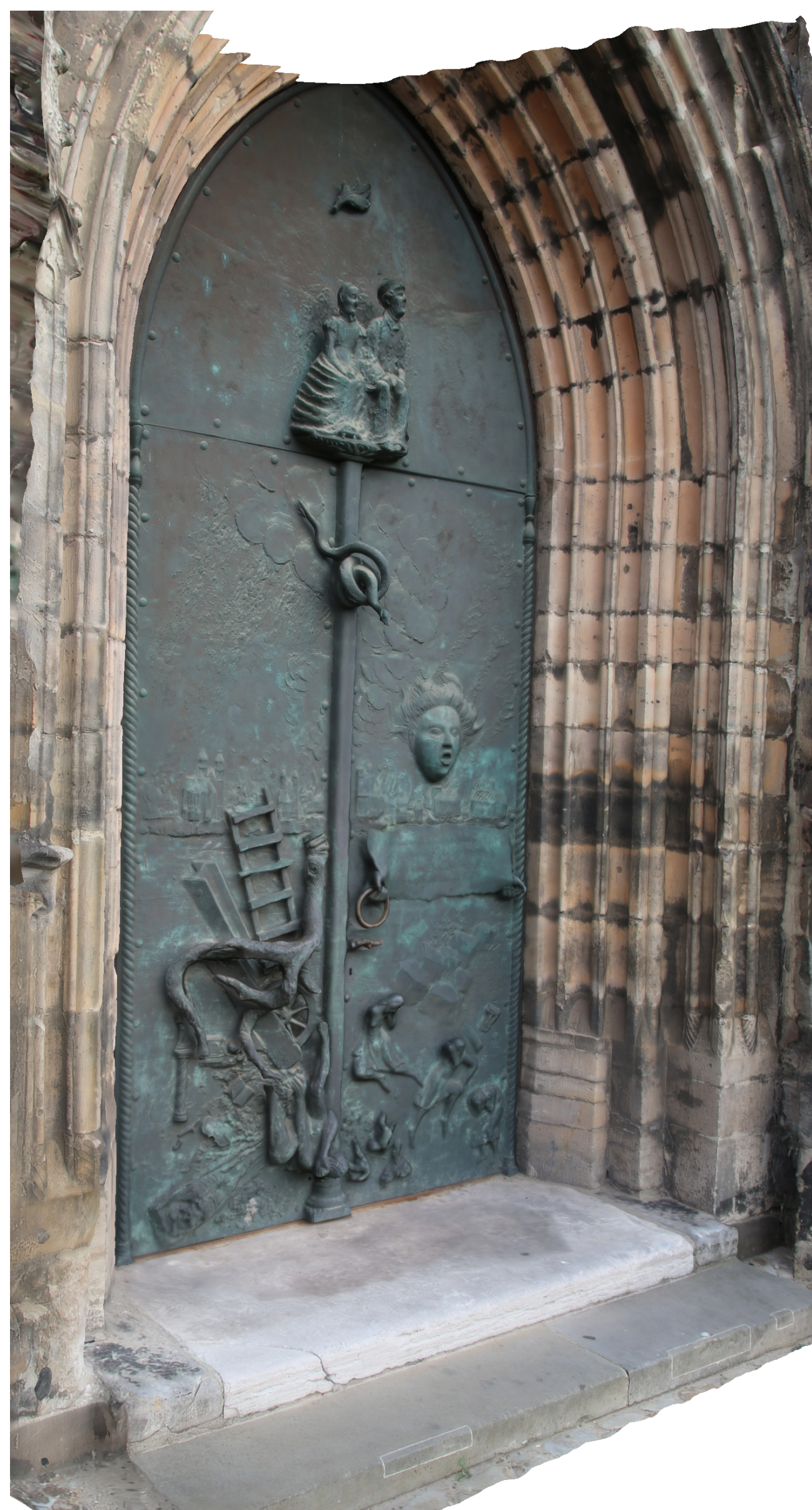
Figure 2. Door of a 8th century cathedral door in Magdeburg, Germany. 100 photographs. Note the concave structures such as the coiled snake and limited side access, limiting many scanning technologies.
