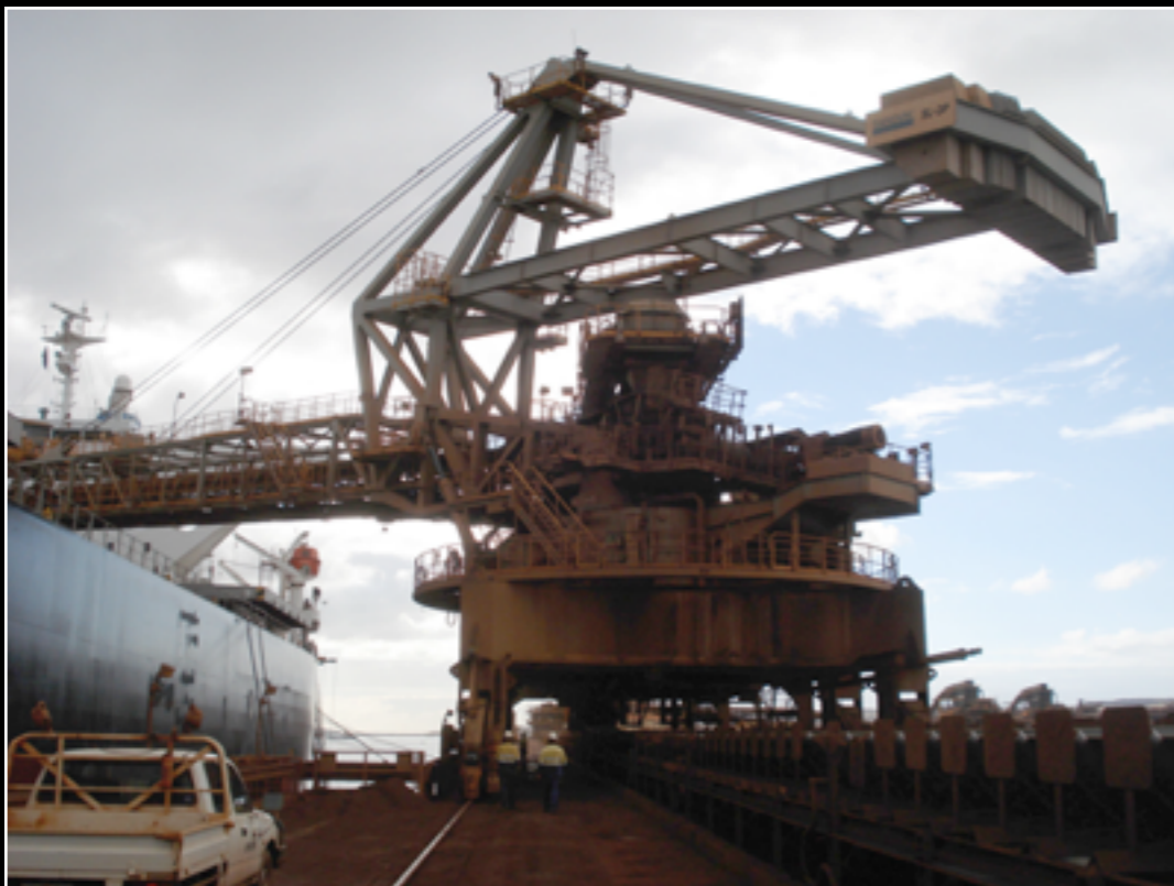
Shiploader, ship on left, iron ore conveyer on left.
