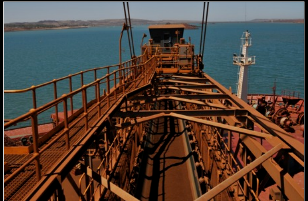
Loading boom over the ship, operator booth at the end.
