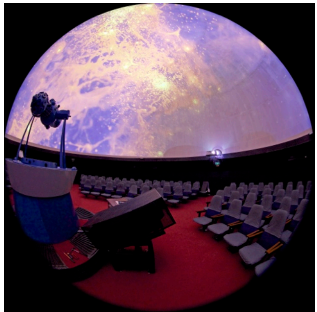
Interior showing Zeiss star projector and spherical mirror; the spring line for the digital projection slightly raised to avoid a shadow from the Zeiss.
