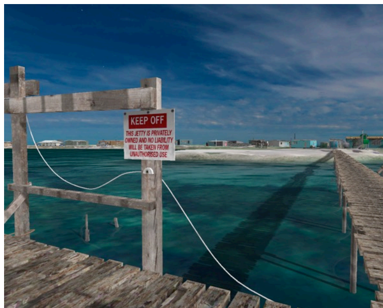
Main jetty entry point
